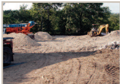
Groundwork is underway on the lodge.
